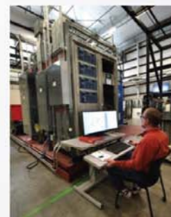
Integrated Energy Systems
